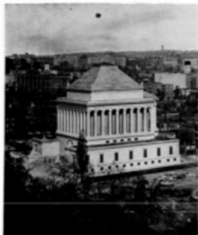
View of Building, Showing Solid Limestone Roof
