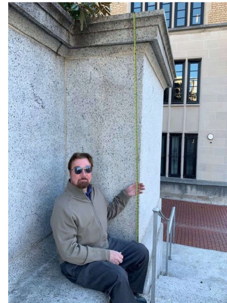
Photo Showing 7'8" Measurement of Granite Wall And Stone Column Above Concrete Platform
